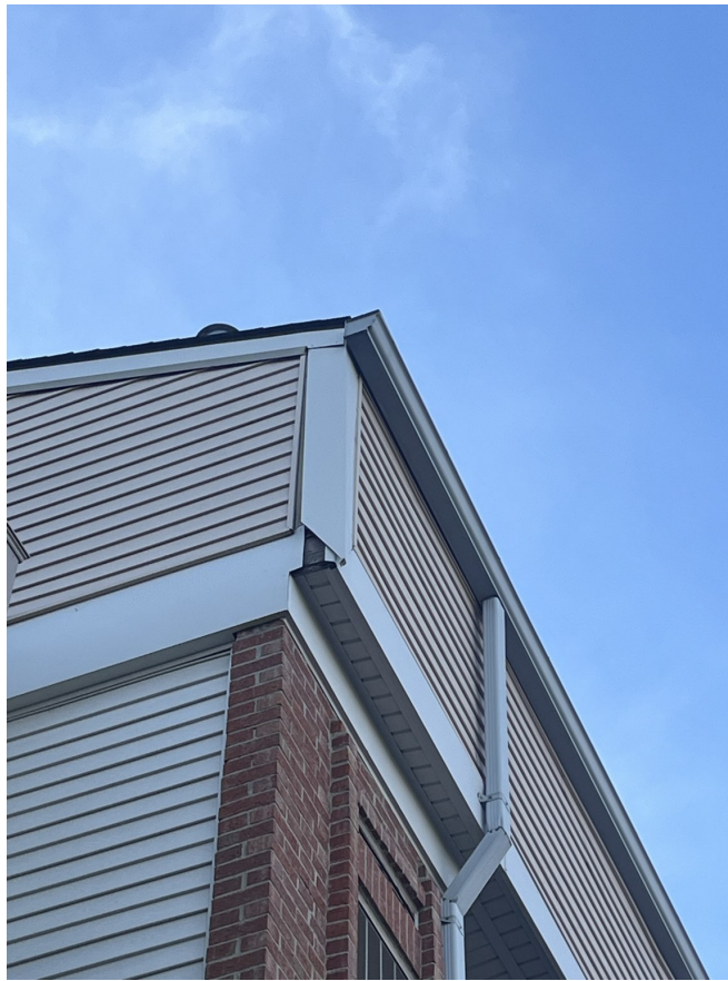
Aluminum trim replacement
