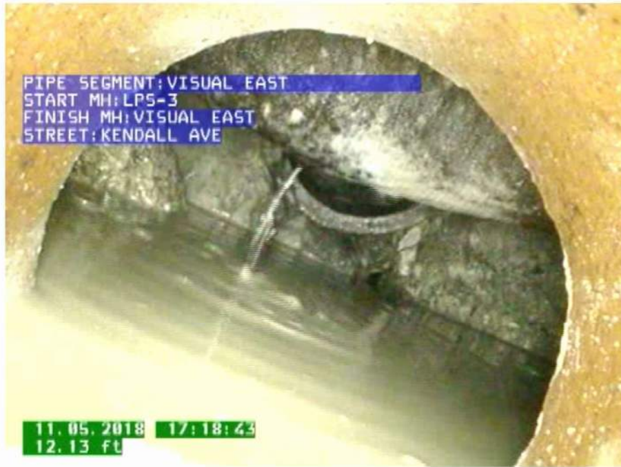
Figure 3 : 2018 CCTV - Visual East of Pipe from Manhole LPS-0-3
