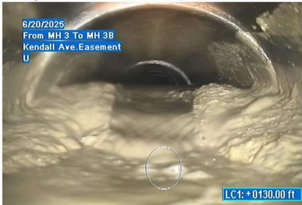
Figure 5: 2025 CCTV - Visual North of Pipe from Manhole LPS-0-5
