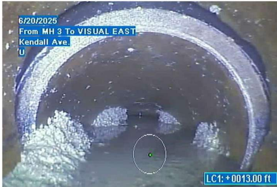
Figure 4: 2025 CCTV - Visual East of Pipe from Manhole LPS-0-3
