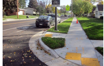
2: An example of a sidewalk that offers both a curb ramp and warning strips.
