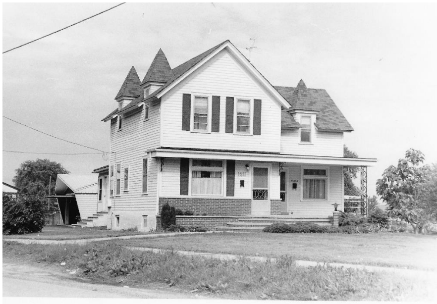
Charles Klein House, Utica Road at Klein
