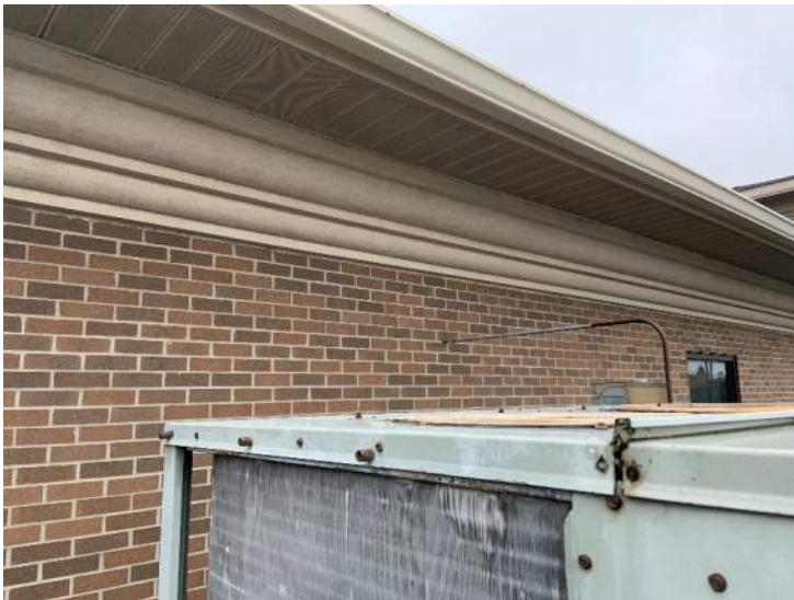
Photo 6: Overhang located above RTU-4
