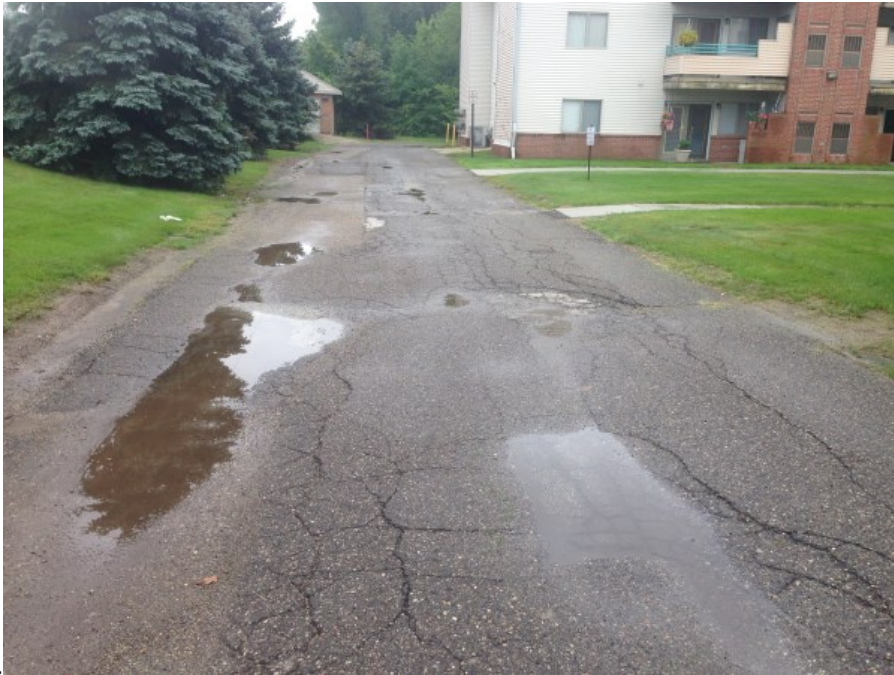
Photograph No. 3: Moderate to high severity fatigue cracking with pavement rutting and standing water near boring B-3. View to the south.
