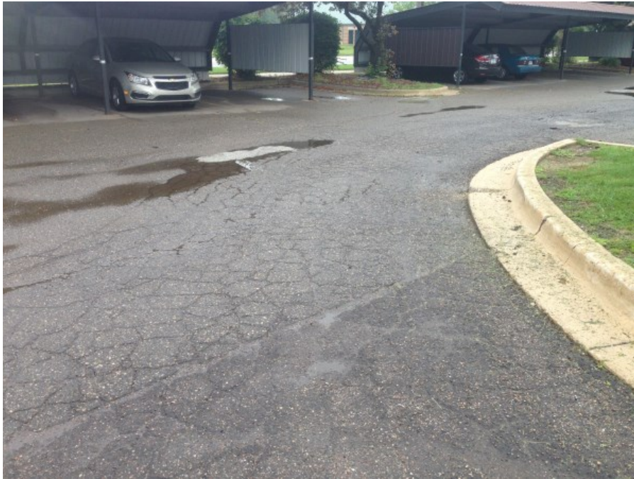
Photograph No. 1: Moderate to high severity fatigue cracking with standing water near boring B-1. View to the northeast.
