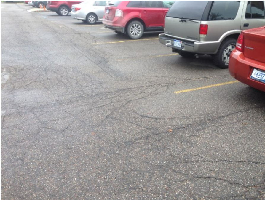
Photograph No. 5: Moderate to high severity fatigue cracking near boring B-7. View to the north.
