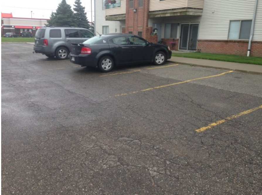
Photograph No. 2: Moderate to high severity fatigue cracking near boring B-2. View to the southeast.
