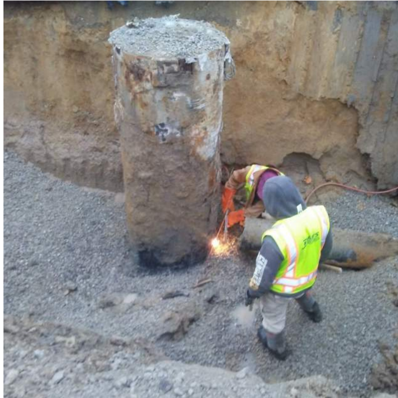
Figure 3.2-4 2016 Collapse – Removing the Casing to Permit Water Main Extension
