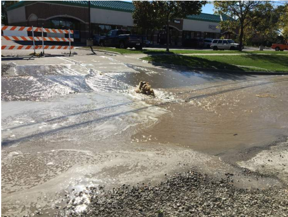
Figure 3.2-2 2016 Collapse – Water Main Break October 16, 2017
