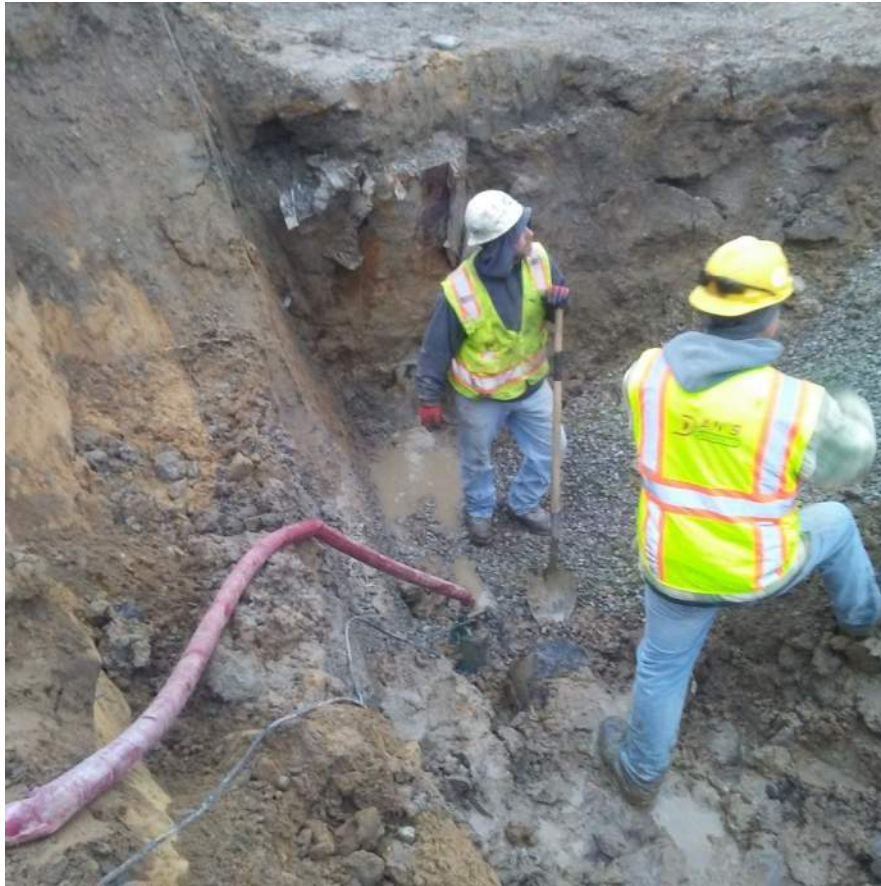
Figure 3.2-3 2016 Collapse – Existing Water Main Open Pipe
