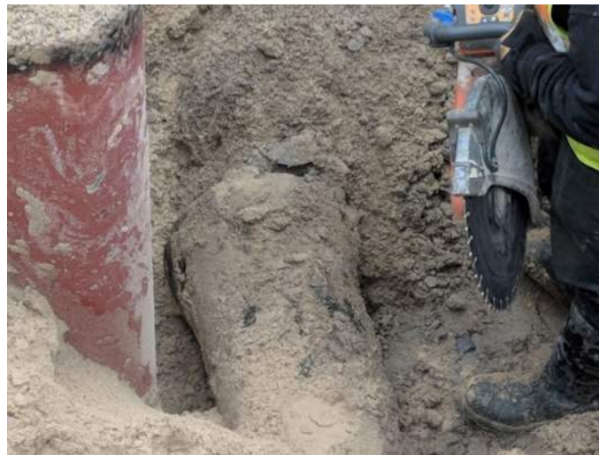
Figure 4.0-2 2019 Break – Termination of Water Main
