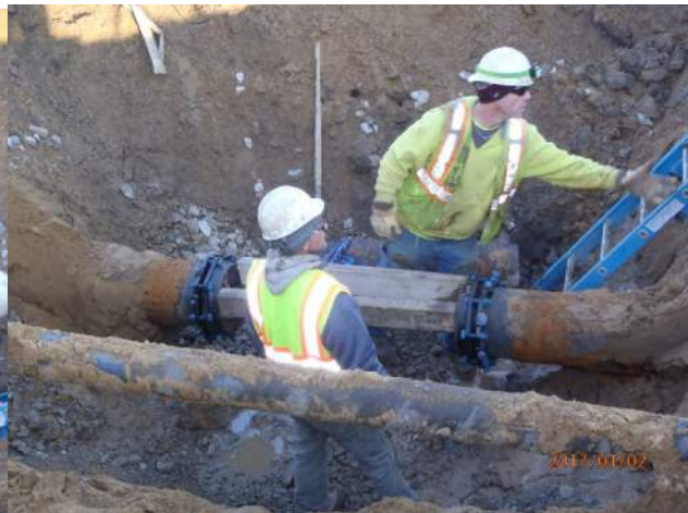
Figure 3.1-5 2016 Collapse – Both Ends Capped
